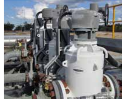
6 x 200 mm, 100bar ash lines, Electric Actuation
