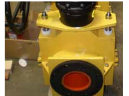
Lime Dosing Manual Pinch Valves
