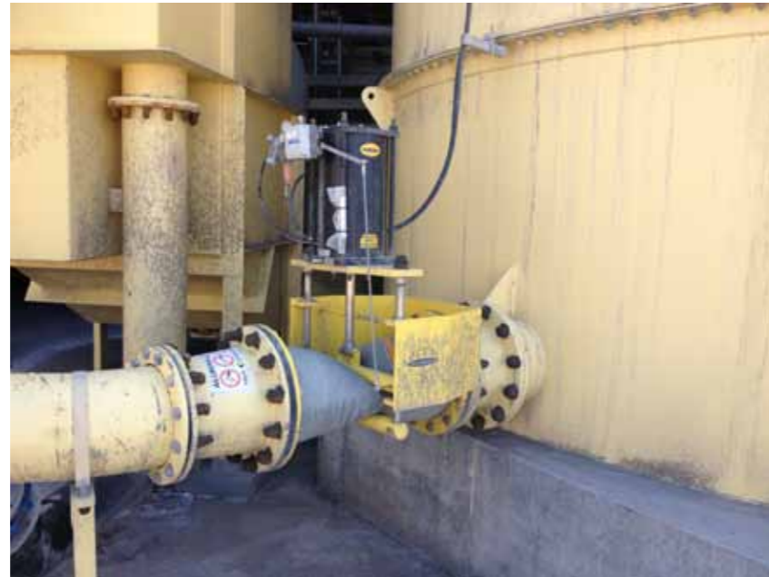
Tank level control valve - smooth flow deflection
