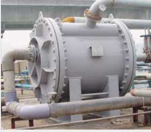
Waste Water Cooler
