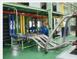
■ Pilot Testing Room
