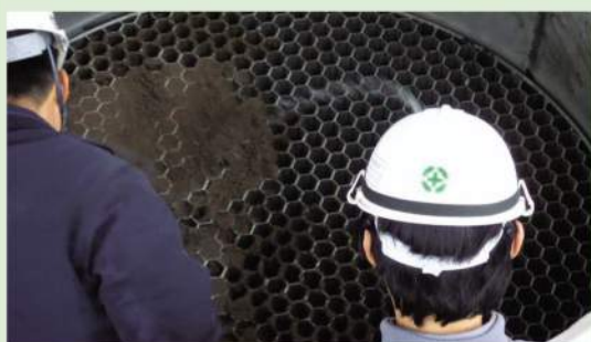
CATALYST CHARGE WORKS
