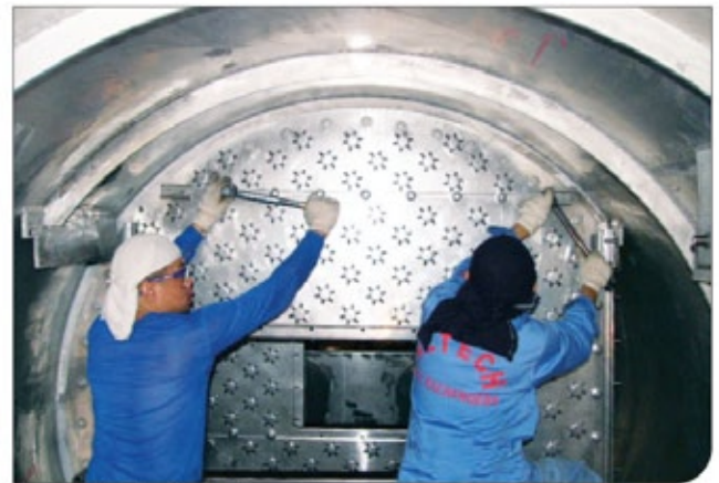
Tray installation inside the column.
