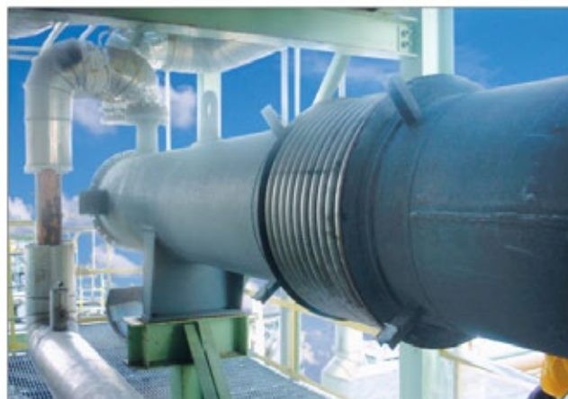
Steam superheater equipped with expansion bellow.
