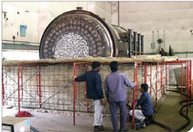
Insitu furnace for PWHT of Waste Heat Boiler.
