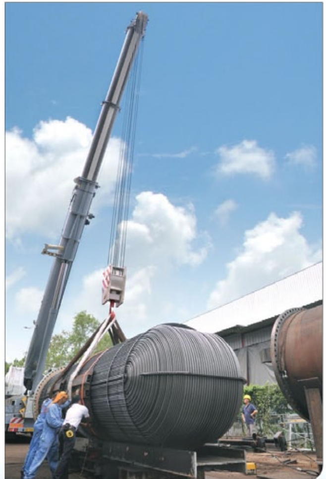
Insertion of 70 tons U-bundle into shell.
