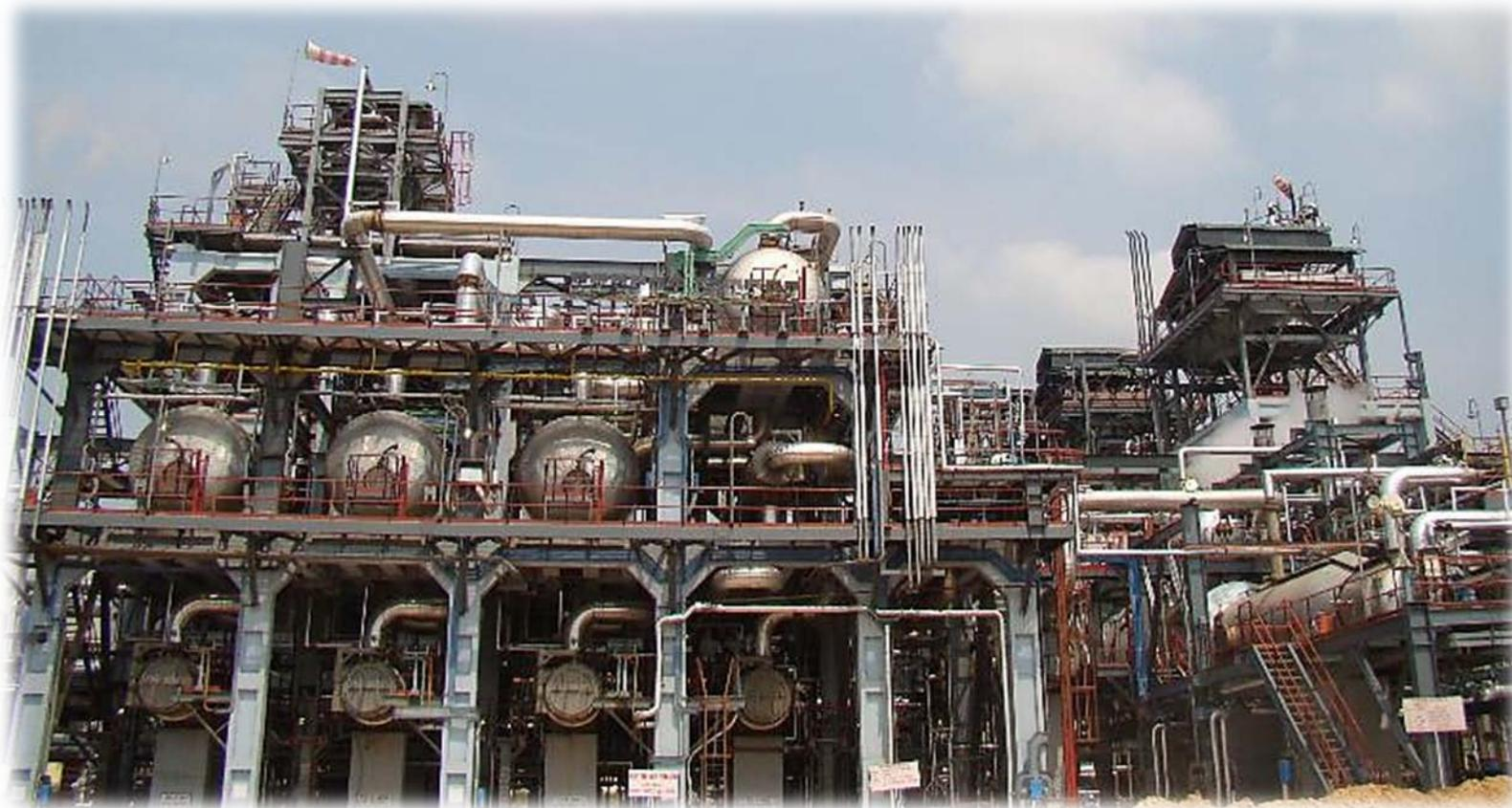
Claus Furnace with Waste Heat Boiler and Sulphur Condensers for BPCL, India
