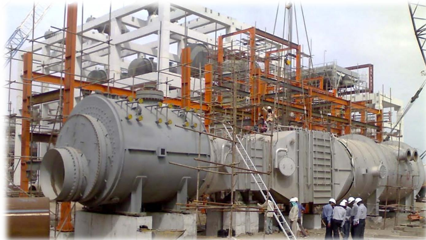
Incinerator Furnace with Superheater & Waste Heat Boiler for ESSAR, India
