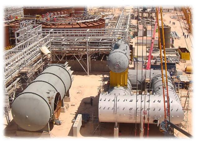
TWIN-Waste Heat Boiler during erection for TIFERT, Tunisia
