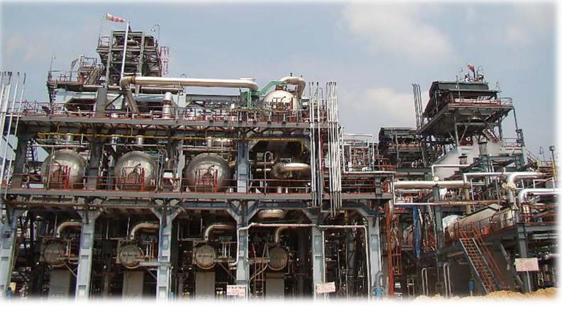
Claus Furnace with Waste Heat Boiler and Sulphur Condensers for BPCL, India
