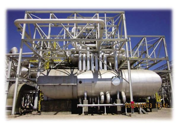
TWIN-Waste Heat Boiler in operation for TIFERT, Tunisia
