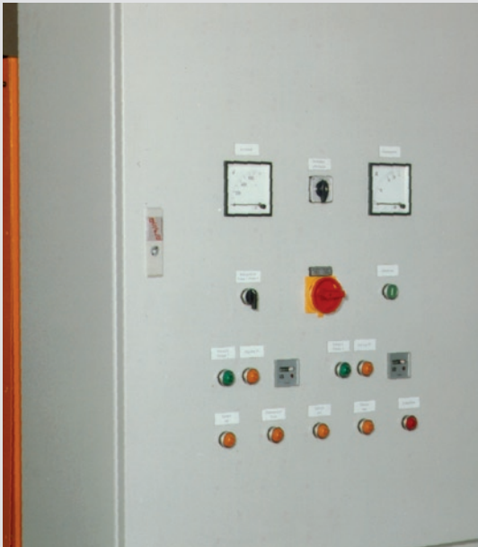
Electro control cabinet (outside sight)
